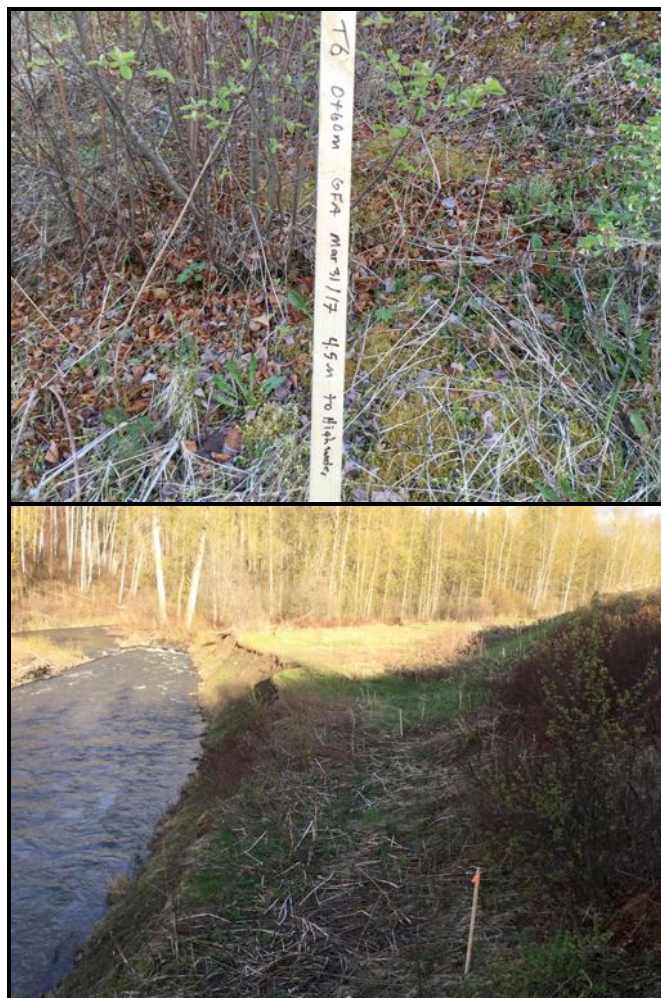
Figure 11: Stake-out area to measure rate of erosion of the Kitwanga River bank adjacent to the Gitanyow Totem Pole and Historical Museum site. On March 31 st , 2017, stakes were placed 3m from the sloughing bank at 10m intervals.
