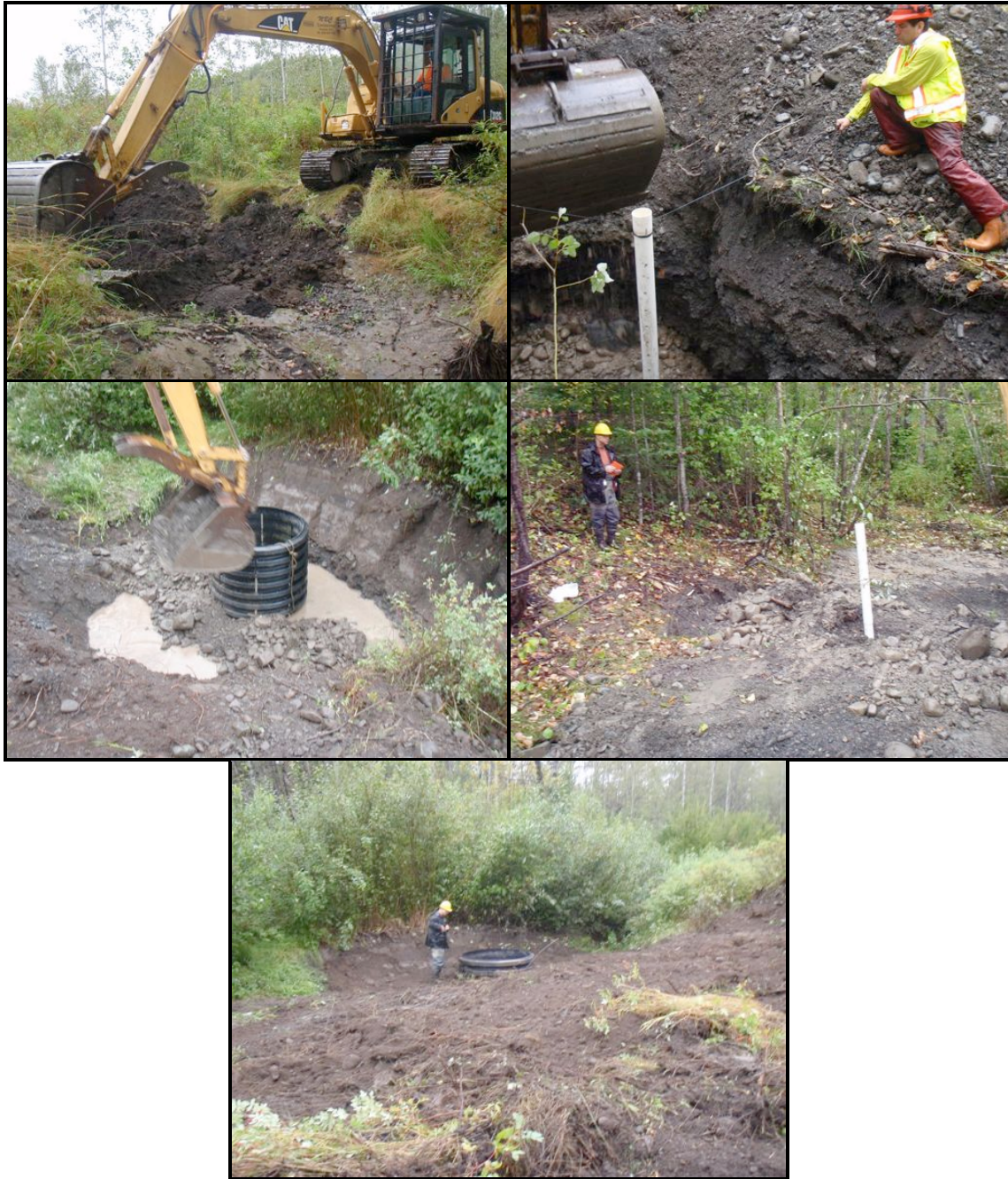
Figure 5: Photo Series showing examples of test and refuge pipes installation on August 30, 2016: pit excavation (top left), test pipe installation (top right), refuge pipe installation (middle left), completed test pipe installation (middle right), and completed refuge pipe installation (bottom).
