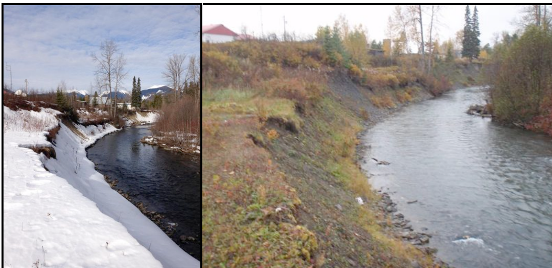
Figure 10: Eroding Kitwanga River bank adjacent to the Gitanyow Totem Pole and Historical Museum site.
