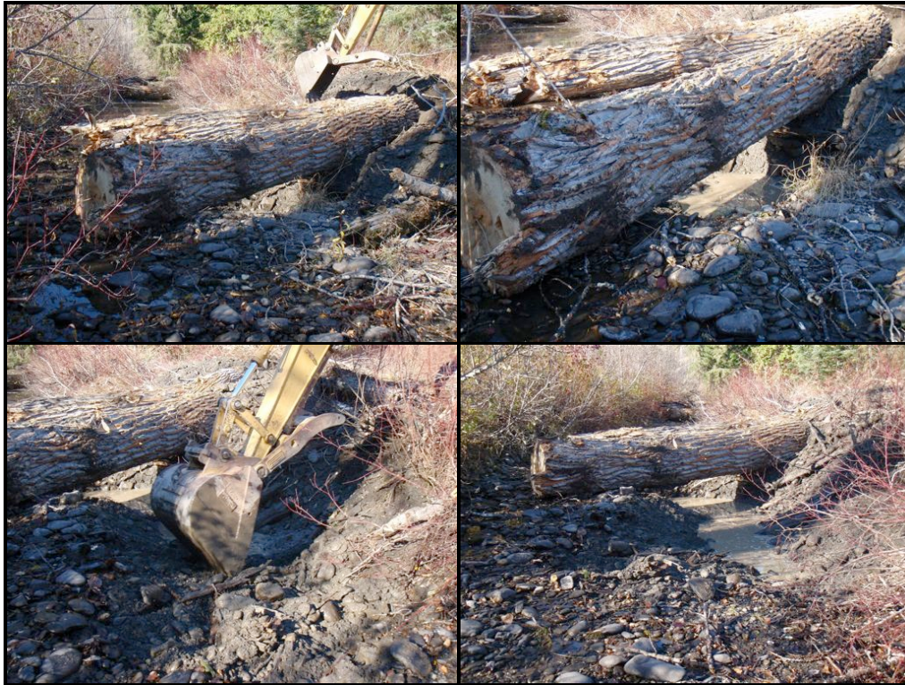
Figure 16: Photo Series showing the installation of the middle LWD cluster on October 11, 2016.
