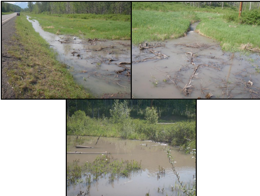
Figure 2: Task 1 Overflow – Annual runoff down Hwy 37N ditch (left); source of overflow over abandoned beaver dam (right) and abandoned beaver dam (lower middle). Photo taken by GFA on May 25 th , 2015.
