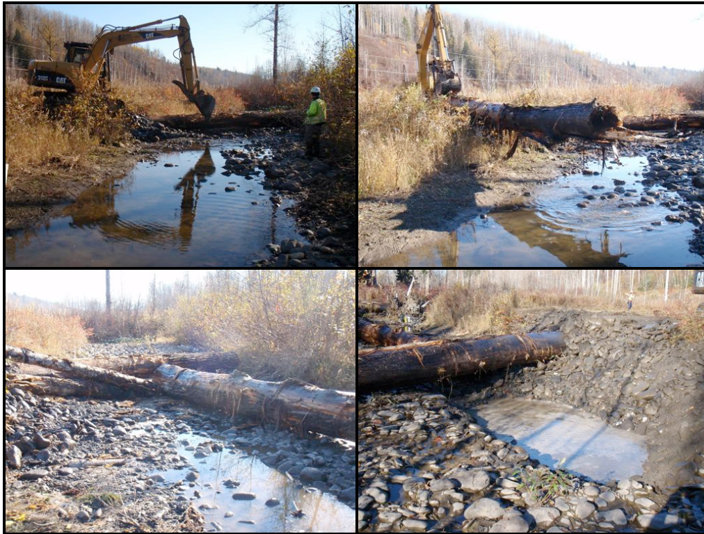
Figure 15: Photo Series showing the installation of the downstream LWD cluster on October 11, 2016.
